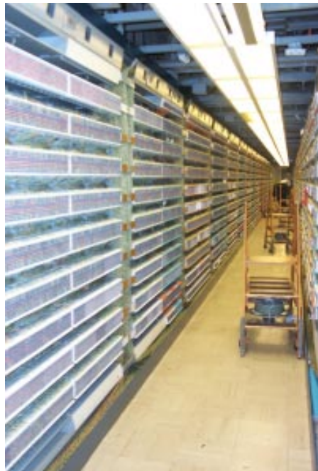
This is the front of the distribution frame where the copper pairs are connected one-by-one to the Central Office switch.
