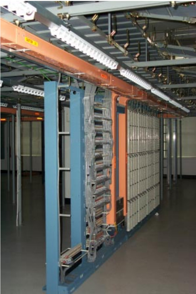
This is bank of DSL multiplexers. Each box (there are three in each of these racks) provides 48 DSL circuits. DSL must be provided end-to-end over a copper pair.
