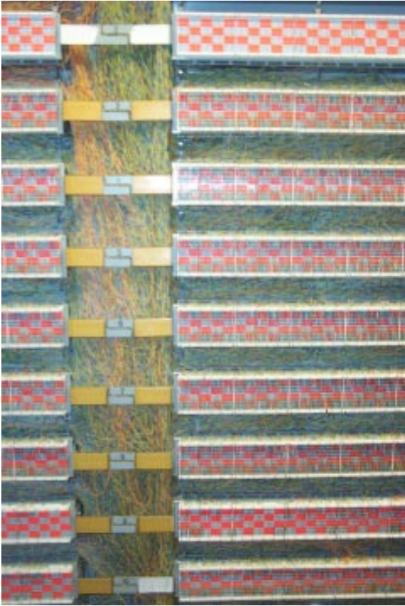
This is the front of the distribution frame where the copper pairs are connected one-by-one to the Central Office switch.
