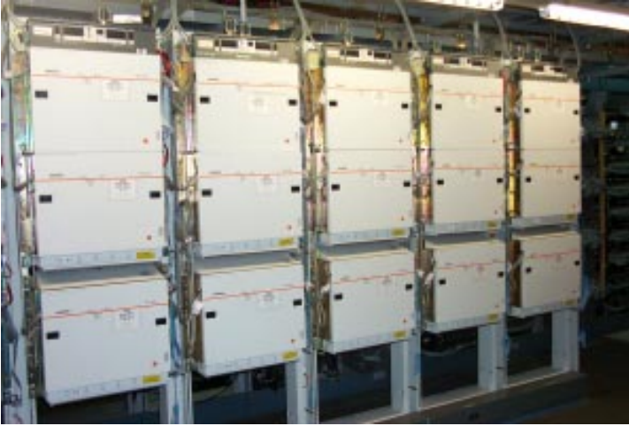
This is bank of DSL multiplexers. Each box (there are three in each of these racks) provides 48 DSL circuits. DSL must be provided end-to-end over a copper pair.
