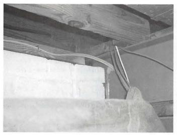
Fig. 3a, 3b: The holes drilled in the floor emerged in a hard-to-reach area of the unfinished area of the basement, requiring barbeque tongs to retrieve the wires once they were pushed through.
