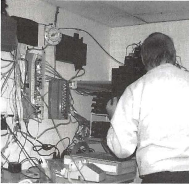
*Dave Weikert restacks modems in the TCS Room. Across the top, from left to right, is a telephone company box, an Ascend router, a round thermometer, and a TribeStar LocalTalk to Ethernet switch. Below these are a network patch panel and a telephone patch panel.*
